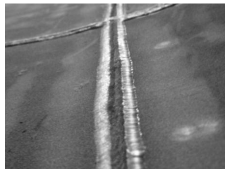
Figure 8: weld repair below tray No. 14
