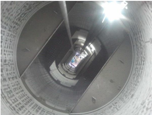
Figure 7: work in progress inside the reactor
