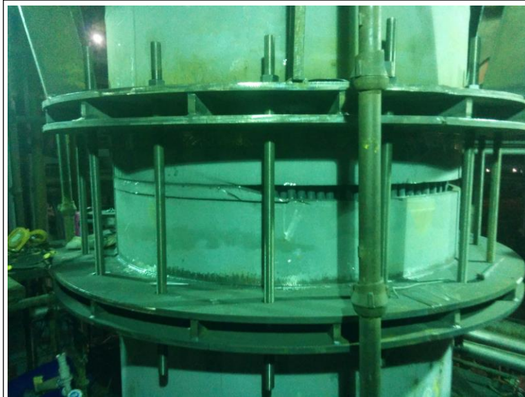
Figure 10: cutting the shell
